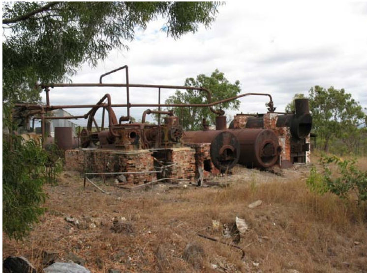
Figure 7: Boilers at the Tyrconnel mine
