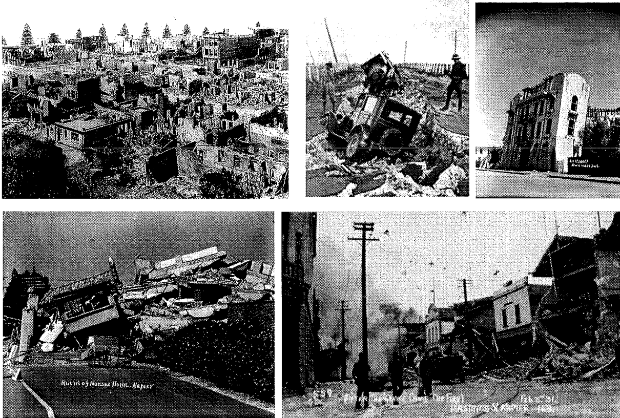
1931 Napier Earthquake damage
